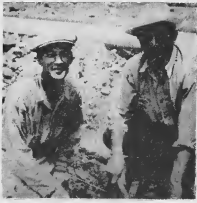
Putting up the new Light Oils Training Building is quite a job and these two messes took for a moment as the cameraman takes their picture.
